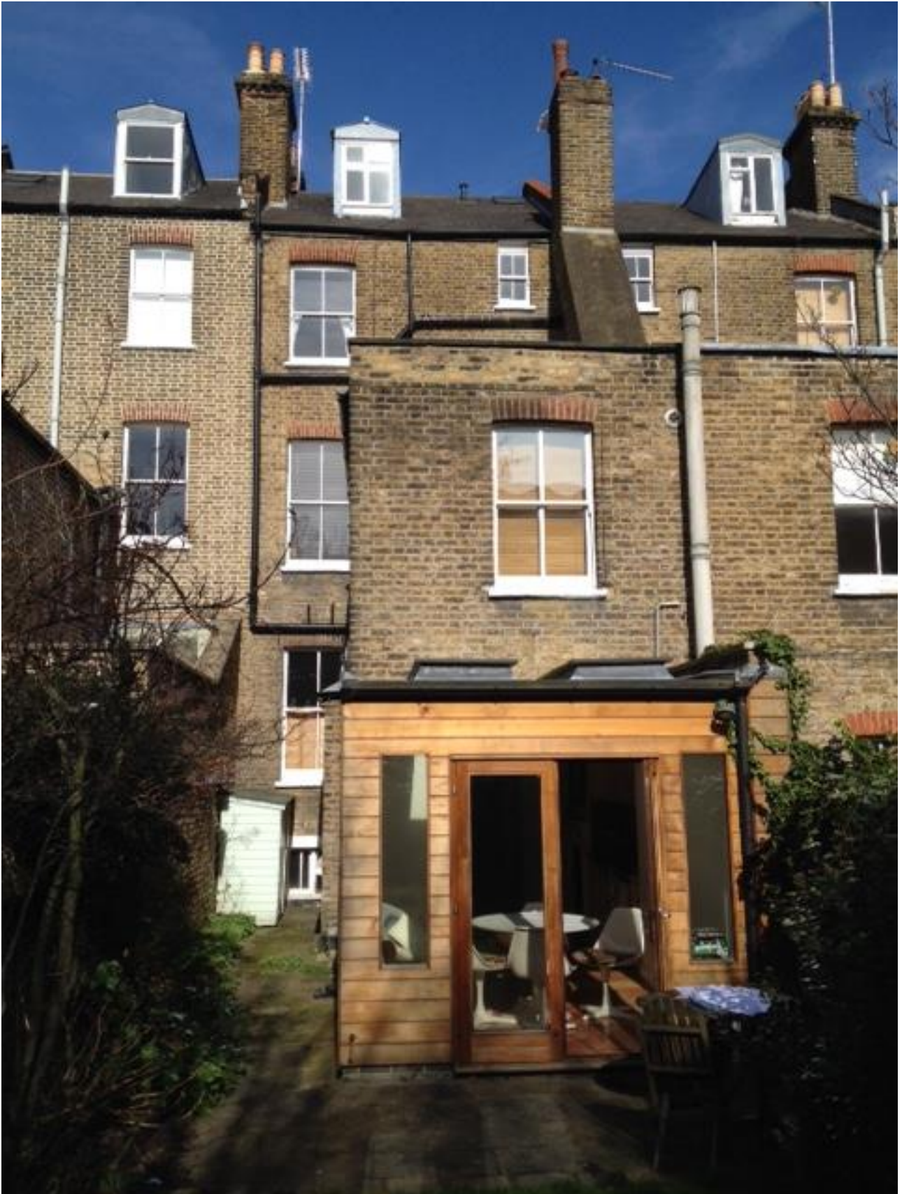
Image 3 – View of Rear Elevation
