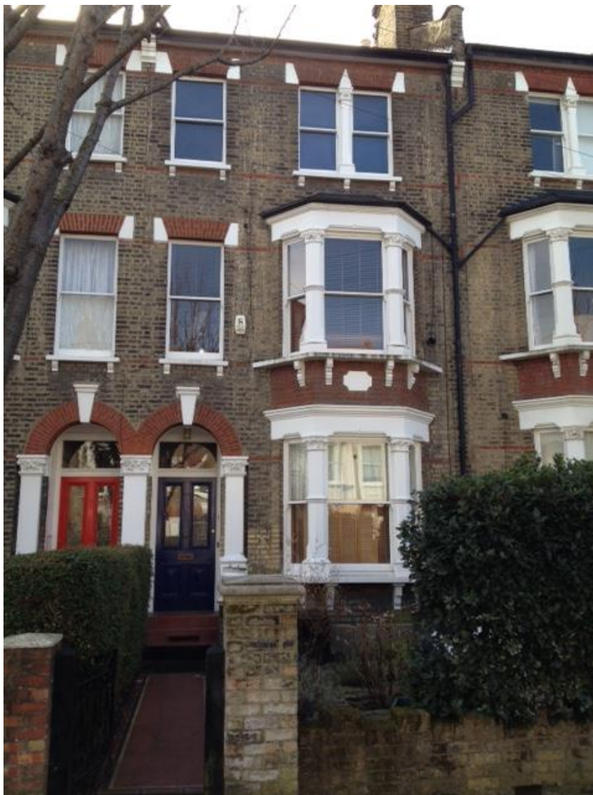
Image 2 - View of front elevation
